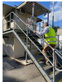
Stair access at winery or at supplier
